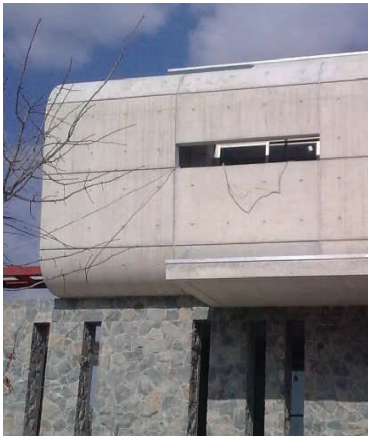
A futuristic private residence under construction — featuring an inclined fair-faced wall section.
