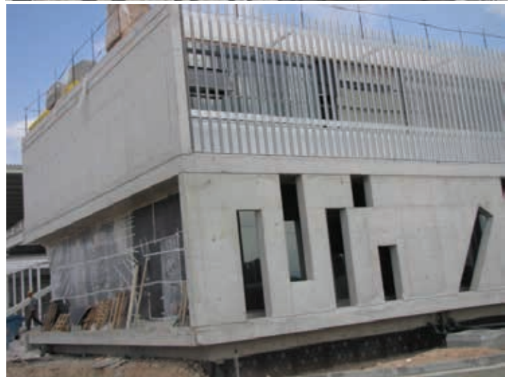
A section of a new extension to a private school under construction — fair-faced concrete is used throughout.
